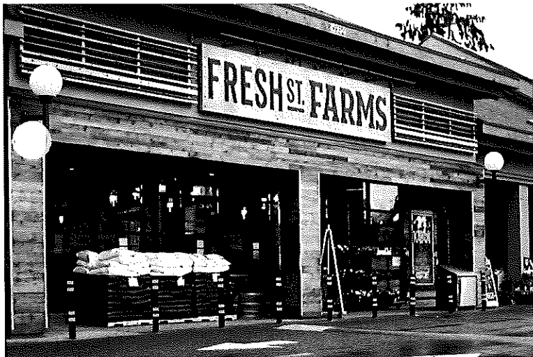
Exposed Wood and Attractive Architecture Elements
